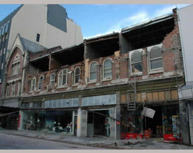
Figure 10 Lucks building, 751 Colombo street and commercial building, 753 - 759 Colombo Street after the 2011 earthquake (and clean up - note all the bricks from the upper part of the second story and parapet walls have been removed.
