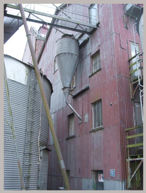
Figure 4 This wall has made its way on to Tellynott. This mill was in Ashburton, but sadly, succumbed to fire a few years ago. A lovely example of corrugated iron cladding.
