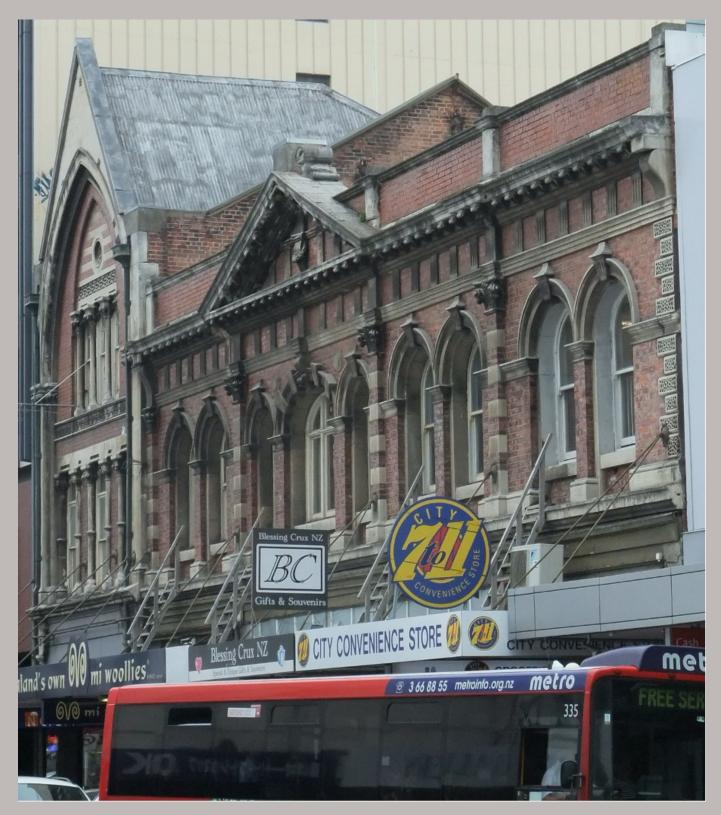
Figure 9 A view from the end giving away a few secretes. Notice the roof is clad in wrinkly tin with a gable behind the façade, but a hip at the back. Also, the tall gable parapet wall at the left end of the left structure. Perhaps there is a lower gable roof behind there.
